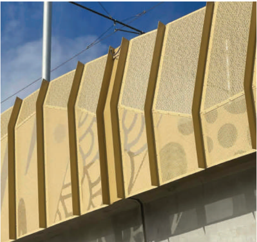
AUD- Tram Grade Separation Project
